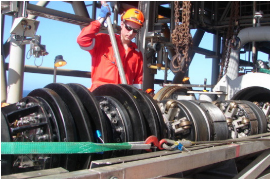
Preloading SmartPlug® tool into the pig launcher.
