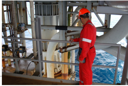
Isolation tool set in the riser.
