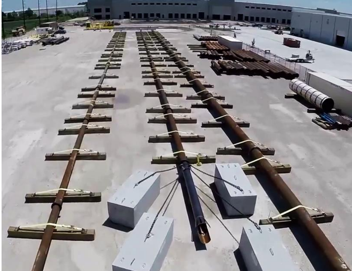
PRCI Technology Development Center Pull-Test Facility. Image © PRCI 2015
