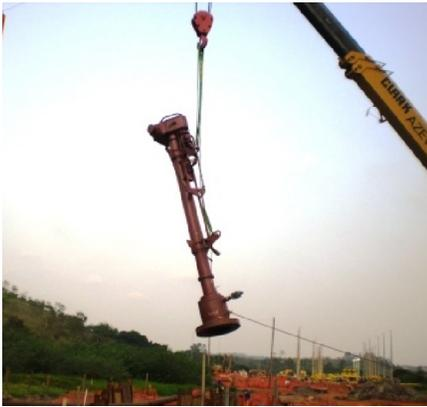
Special plugging head used due to pipeline's pressure capacity of up to 70 bar.
