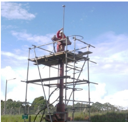
TDW Hot Tapping & Plugging Services enables repairs without environmental damage.
