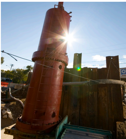
World's largest plugging operation to date: 102" with 60" by-pass.
